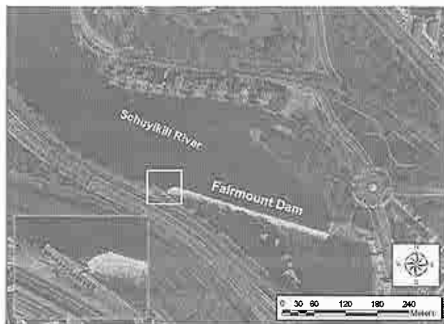
Figure 2. Aerial view of Fairmount Dam and vertical slot fishway (left insert) located on the west bank of the Schuylkill River at river km 13.6, Philadelphia, Pennsylvania.
