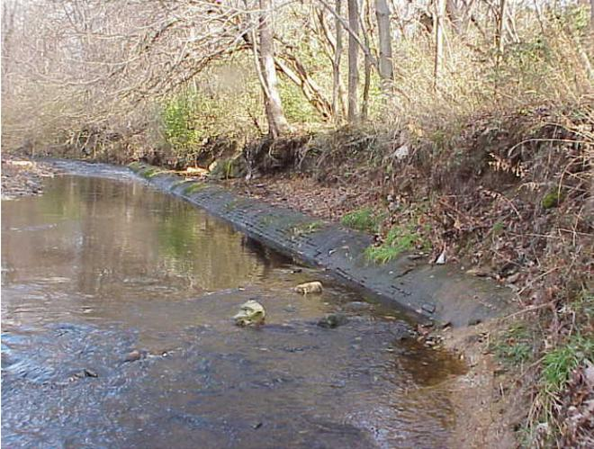
**Figure 1-5 Marshall Road Pre-Restoration (Note Exposed Interceptor)**
